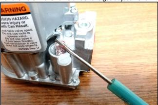
10. Install the new spring and gas adjustment screw in the gas valve. Turn the screw clockwise all the way in until it bottoms out. Then turn the screw out counter-clockwise **5** turns.
